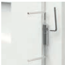
adjustment of 3D adjustable barrel hinges
