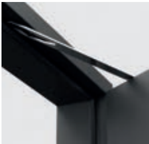
spring loaded door closer
